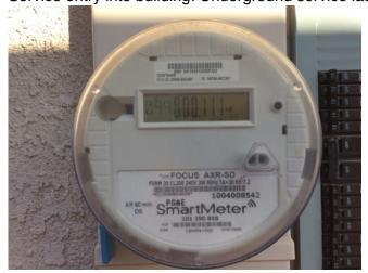
Voltage supplied by utility: 120/240 volts Capacity (available amperage): 125 amperes
