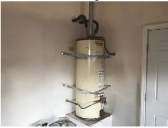
As preventive measures, we recommend that the water heater be equipped with seismic straps and approved flexible gas and water supply connections.
