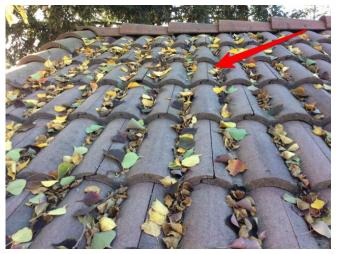
Trees are overhanging the roof. We recommend they be trimmed to prevent debris from accumulating on the roof and to prevent damage by abrasion.
