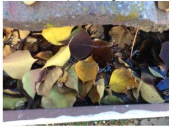
Portions of the gutters were filled with water at the time of this inspection. We recommend all debris be removed and the downspouts be flushed to ensure proper drainage. The condition of the gutters can be better assessed at that time.
