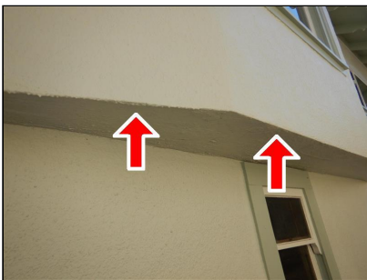
Missing drip edge flashings
