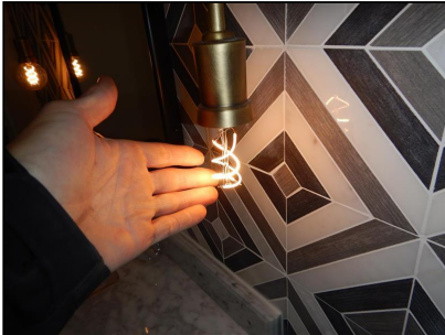
Damaged light bulb
