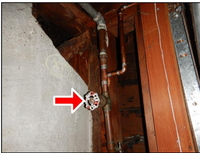
Main water shutoff valve
