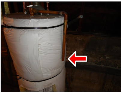
Short discharge pipe
