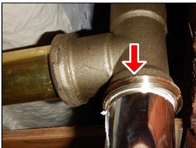
Missing slip joint nut
