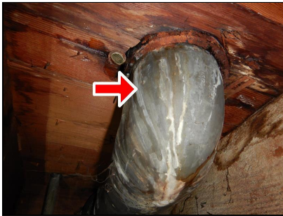
Leaking drain piping
