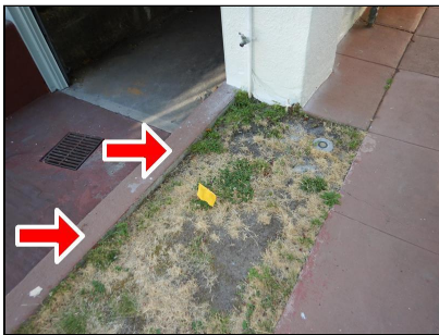
Missing guardrail
