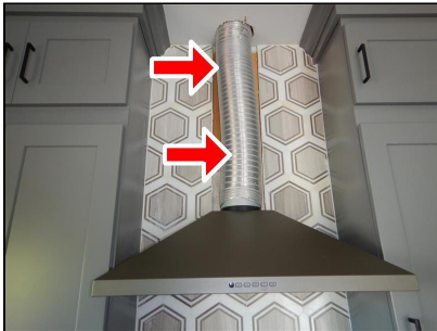
Corrugated kitchen vent
